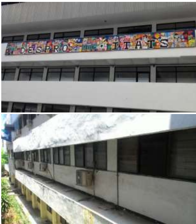
Fig.5: Interior of atrium and windows in the envelope of G-Building ITATS
