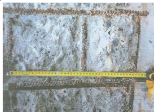
Fig. 3: Reinforced Steel Bar Pull Detection Activities
