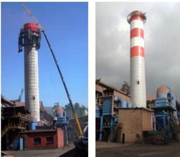
Fig. 9: View of chimney after jacketing and after painting
