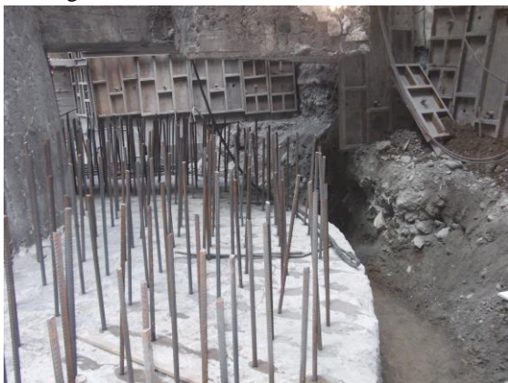
Fig. 6: Anchor works in chimney foundation
