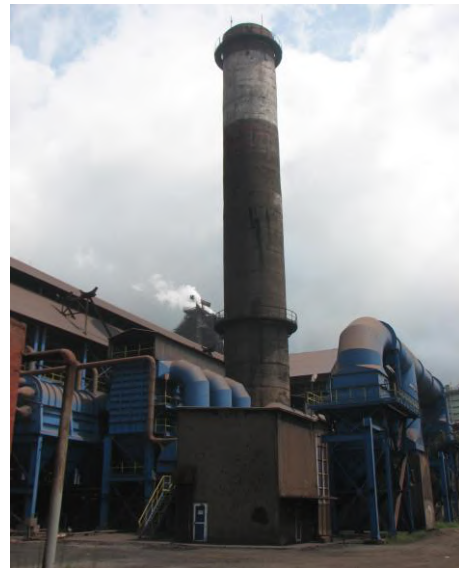
Fig. 1: General view of the chimney
