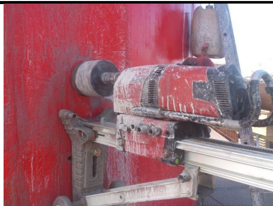
Fig. 4: Taken concrete samples from chimney
