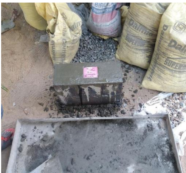
Fig.3.8: Concrete Poured in Deep Beam Mould and leveled
