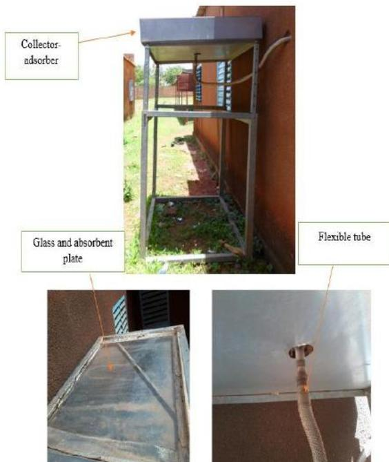
Fig.3. Detailed photograph of the collector-adsorber.
