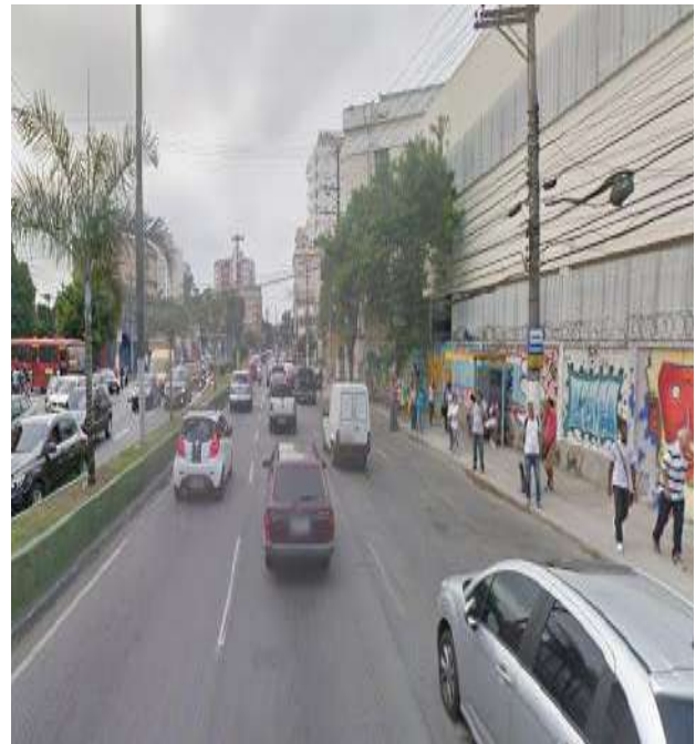
Fig. 5 (a) Old bus stop in Marquês do Paraná Avenue near the tunnel Angela Fernandes.
