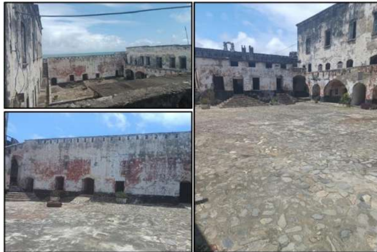
Fig.8. Courtyard within Fort Williams Source: Site investigation by author, 2025.
