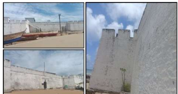
Fig.7. Exterior Walls of Fort Williams Source: Site investigation by author, 2025.
