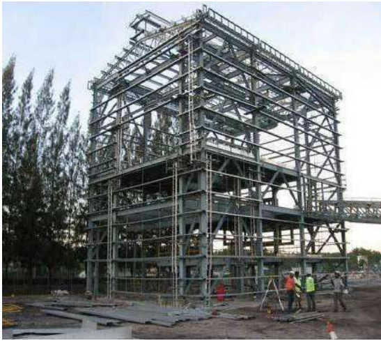
Fig.1: Steel structure installation
