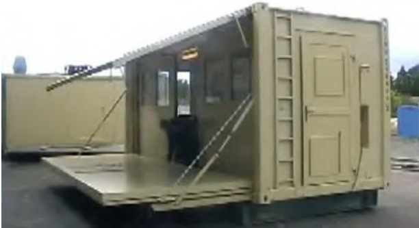
Fig.5 - Foldable structure being assembled
