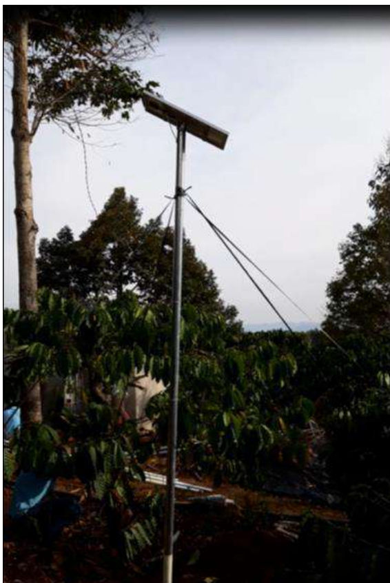
Fig.9. Installing a Pole Mounted Solar Panel
