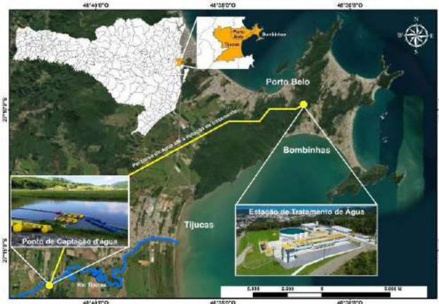
Fig.2: Water intake from Tijucas River to the Zimbros Water Treatment Plant.
