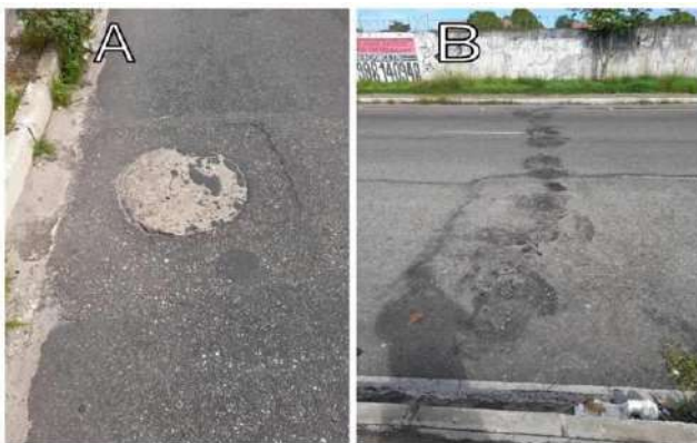
Fig. 8 - (A) Local plastic sinking; (B) Degradation of the ligand.
