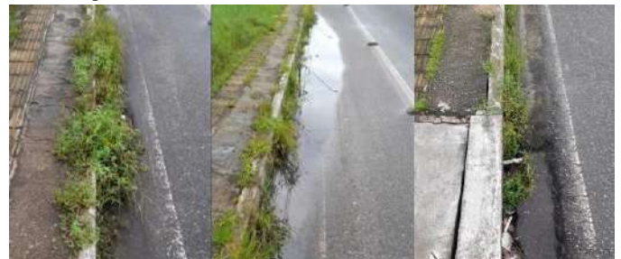
Fig.12 – Gutter silting.
