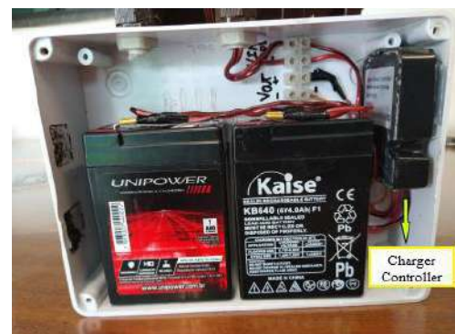
Fig. 11 Mounting the system battery and charge controller.
