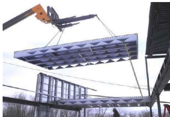
Fig.3: Example of erection of panelized floor.
