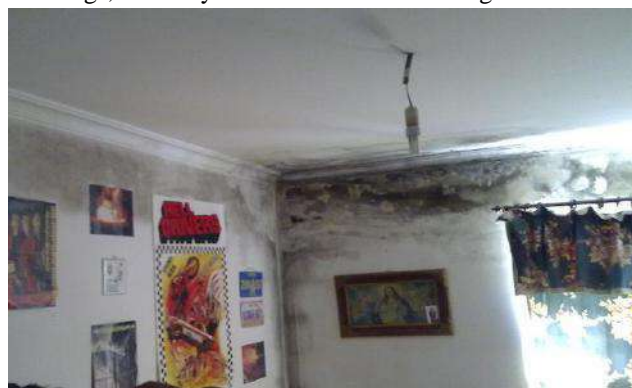
Fig.3: Moisture and mold on walls. Source: Own authorship.
