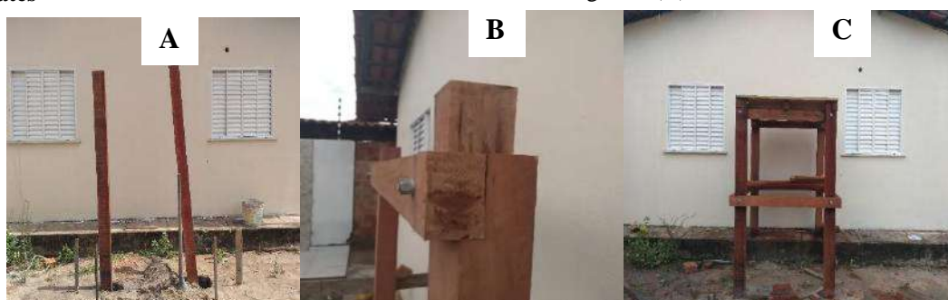
Fig.3: A -Feedback and positioning of the pillars; B - sections for stability; C -ready wooden structure.
