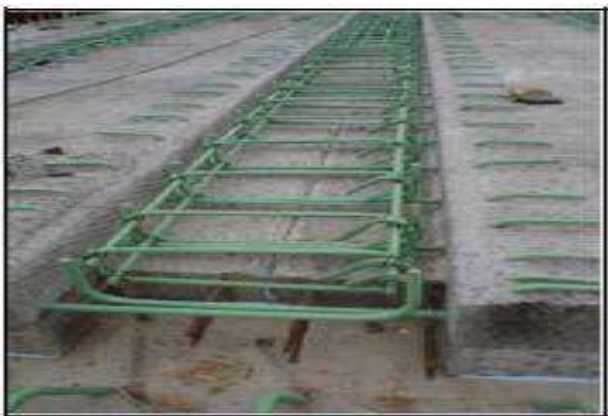
Fig. 1: Closure joints for accelerated bridge construction
