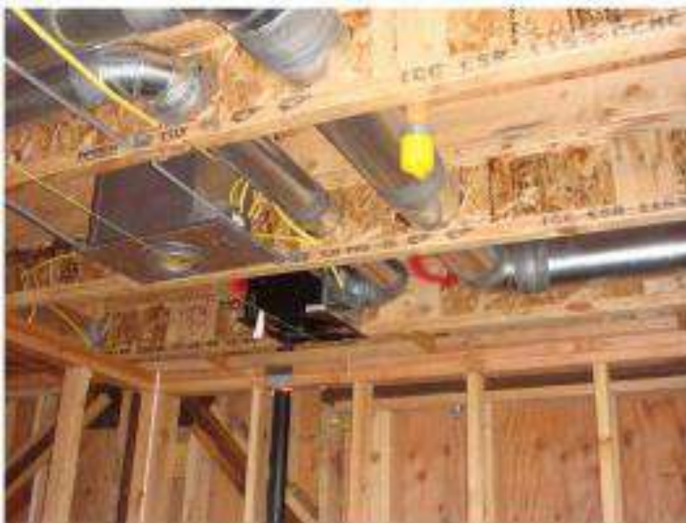
Fig. 5: Examples of Holes In Wood I-Joists, Tiberiu Polocoser, Thomas H. Miller, And Rakesh Gupta, 2013
