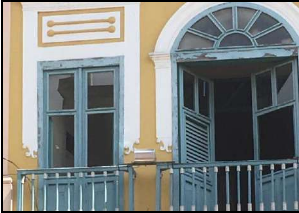
Fig. 9: Wear of the frames
