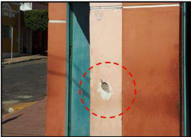
Fig. 4: Plaster detachment
