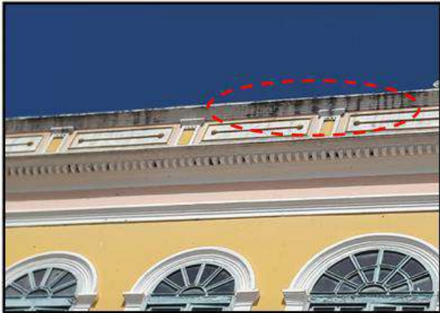
Fig. 6: Surface spots characterized by moisture
