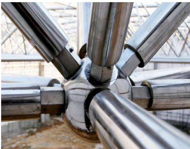
Fig. 1-1: The bolt-ball node joint
