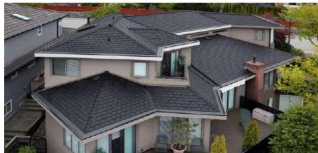
Fig.2: Composite roof of 70% tire.
