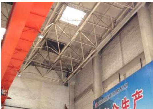
Fig. 3-3: Lower chord bending
