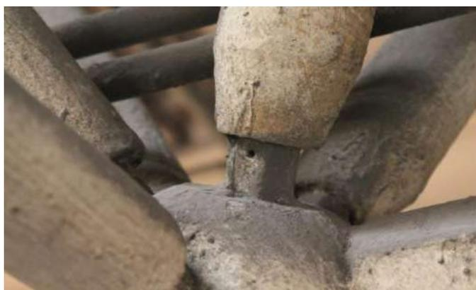
Fig. 3-8: Bolt sleeve pin is missing
