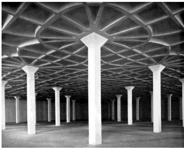
Fig 6.b Pier Luigi Nervi roof
