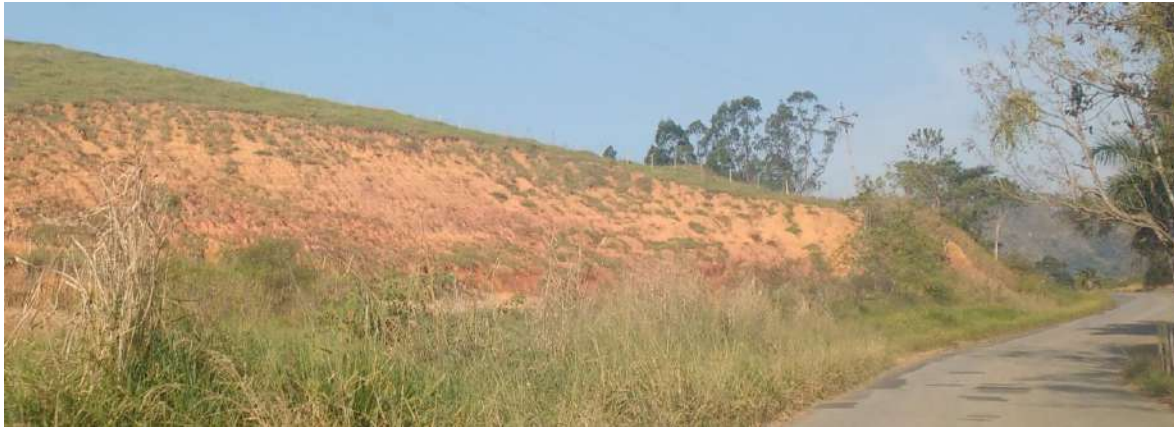
Fig. 6: Erosion in pasture area, in São José community.
