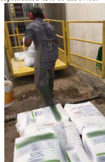
Fig. 4: sacks positioning mp1.
