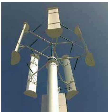
Fig. 2: A VAWT with relatively fixed blade angles
