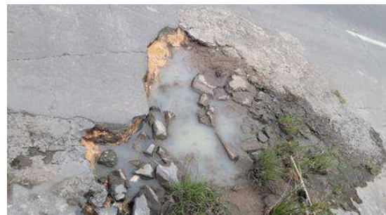
Fig. 20: Pot hole reaching the base, on the pathway (Copyright Images)
