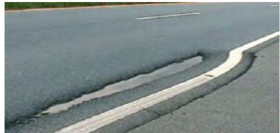
Fig. 10: Slipping (Inova Civil, 2019)
