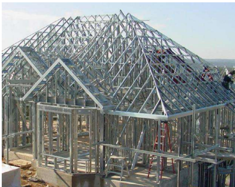
Fig.5: Steel Frame Construction
