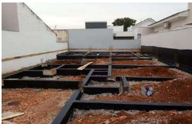
Fig.2: Waterproofed Baldrame Beam.
