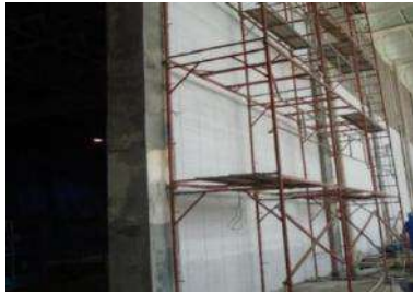
Fig. 7: Scaffolding of the work.
