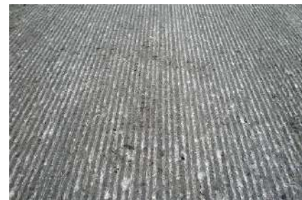
Fig 16 Milling
