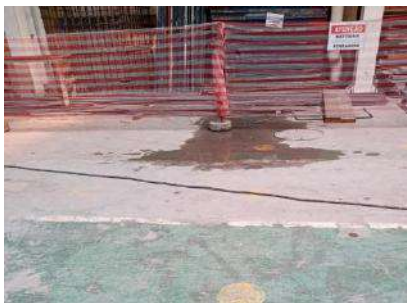
Fig. 8: Electrical cable found in the worksite.
