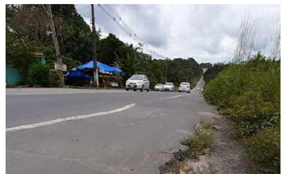
Fig. 26: Sinking (Copyright Images)
