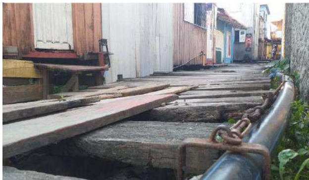
Fig. 6: Aerial Supply Network made with HDPE tube.
