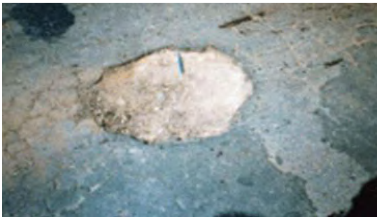
Fig. 13: Pot hole reaching the base (Inova Civil,2019)
