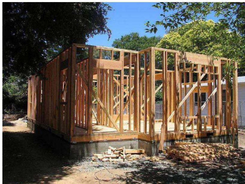
Fig.4: Wood frame construction
