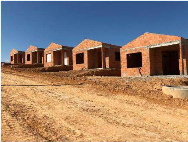
Fig. 6: Houses in structural masonry, Vila Smart Campo Belo, Iranduba, Amazonas.
