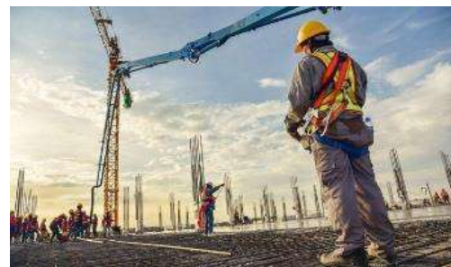
Fig. 1: Construction Site Environment. Font: Correios do MS, 2019.
