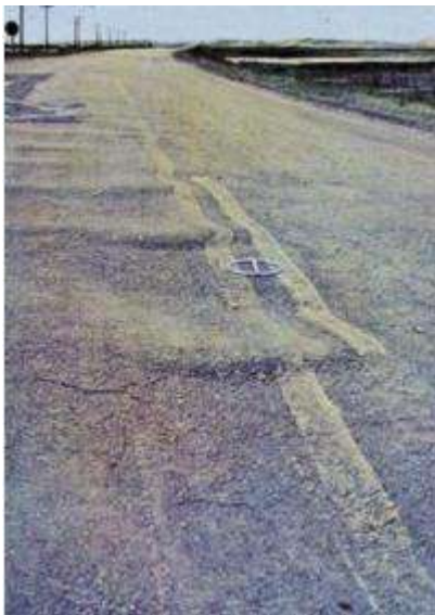
Fig 6 Corrugation example, DNIT (2003)
