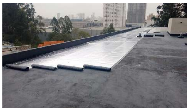
Fig.3: Waterproofing of exposed slab.
