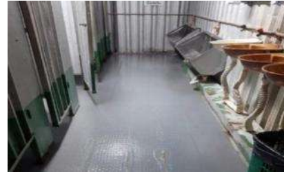
Fig. 5: Sanitary construction site installation
