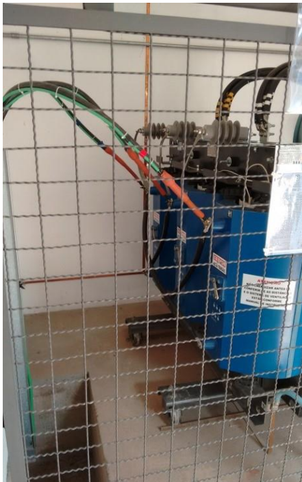
Fig. 1. Dry-type transformer used for the experimental measurements. Source: Authors.
