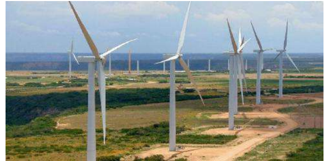
Fig.7: Wind power plant
