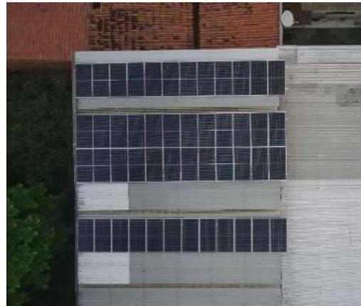
Fig.1: Image of the 19.2 kwp Solar System
