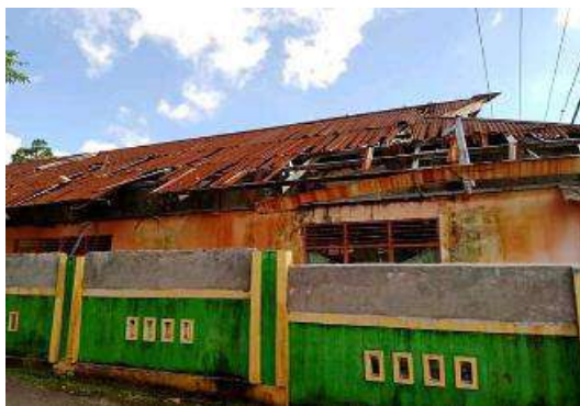
Fig.2 Roof Damage
