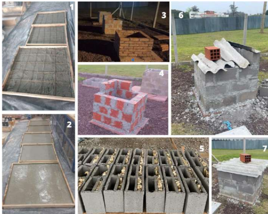
Fig.4 – Building of the prototypes.
