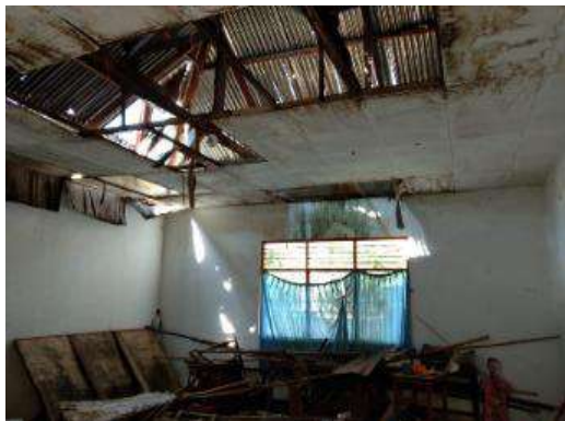
Fig.3 Ceiling damage
