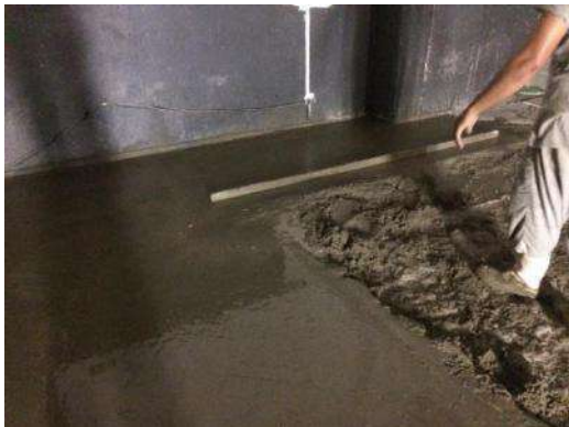
Fig. 5: Leveling with the ruler, Source: Own authorship, 2019.
