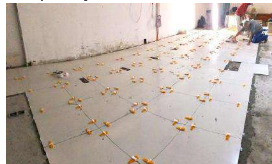
Fig. 7 - Placement of porcelain floor, Source: Own authorship, 2019.
