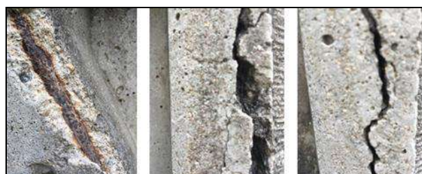
Fig. 8 - Corrosion detail of the of public lighting poles
