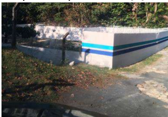
Fig. 6: Sewage treatment station
