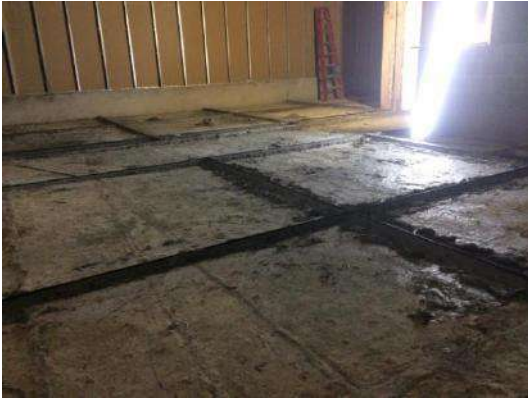
Fig. 4: Fixation of expansion joints, Source: Own authorship, 2019.
