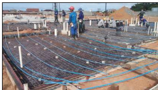
Fig. 5: Placement of chords Source: Own authorship, 2019
