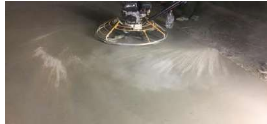
Fig. 6: Floor straightening, Source: Own authorship, 2019.
