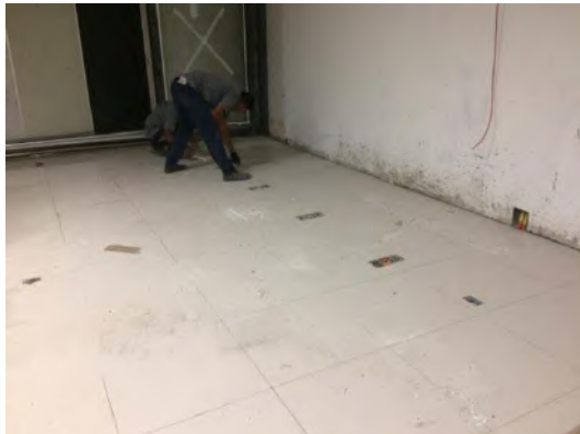
Fig. 8 - Placement of porcelain floor, Source: Own authorship, 2019.
