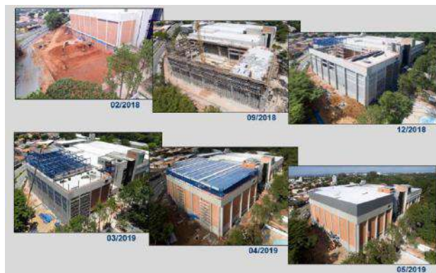
Fig. 9: Evolution of the works on LIT laboratory extension project.
