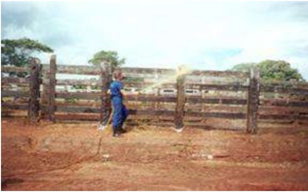
Fig. 12: Cleaning and disinfection work
