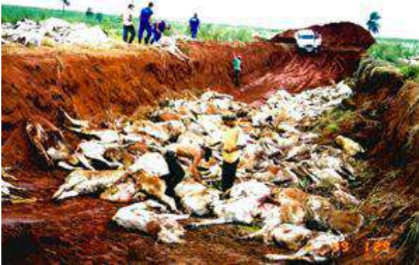
Fig. 6: Work of opening animal carcasses inside the ditch to prevent gas build-up.
