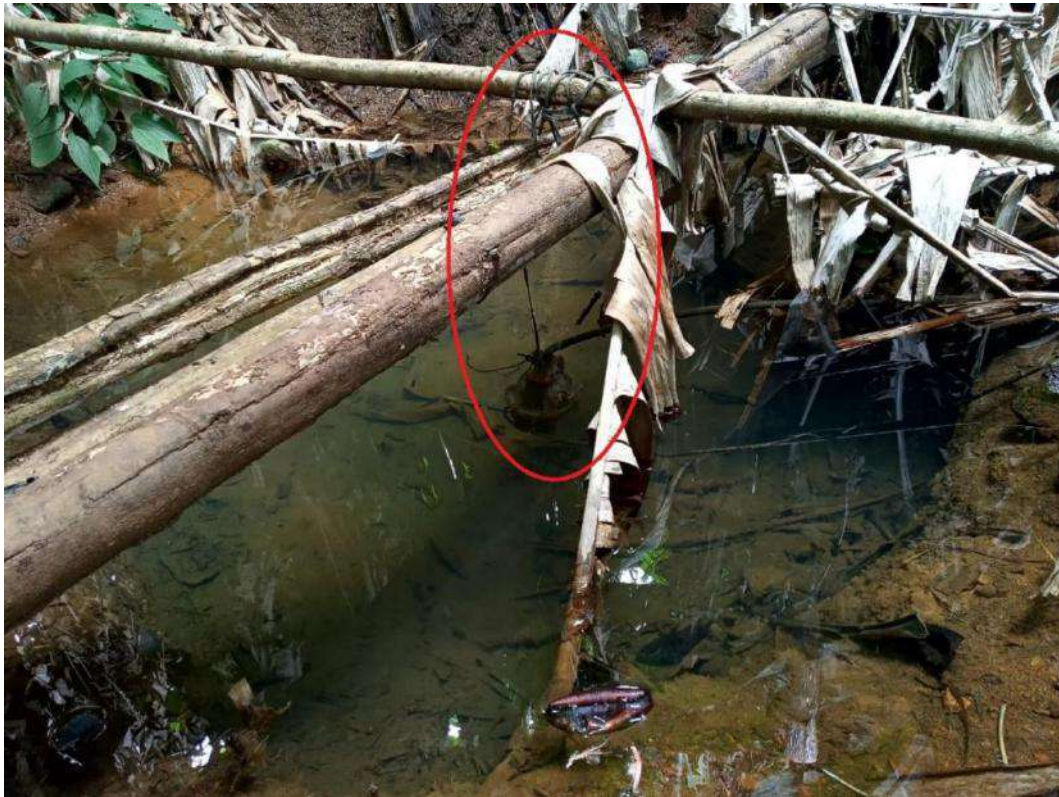
Fig.16: Suction and water holding in P4.
