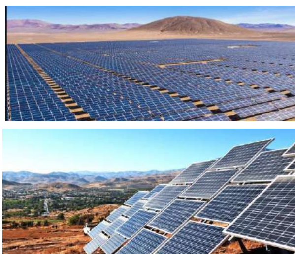
Fig.3: Shown Libya Construction of 100 MW Solar Power Plant in Kufra Town.
