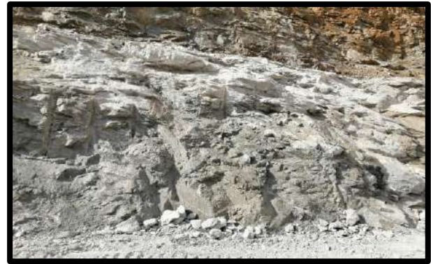
Fig.4.1: Wall Face after Wall Control Blasting
