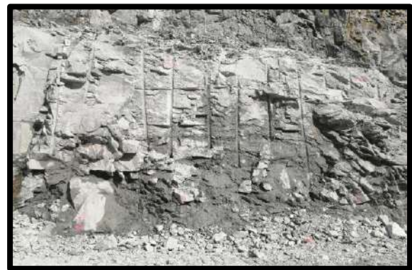
Fig.4.2: Wall Face after Wall Control Blasting
