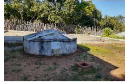
Fig.4: Cistern for rainwater collection and use.
