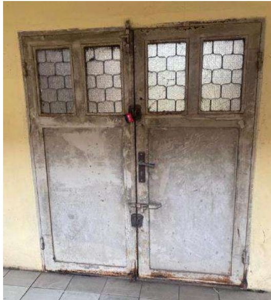
Plate 3: Image showing the fire escape door, brick wall, and escape staircase in the building.
