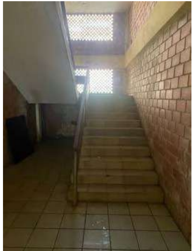
Plate 5: Image of Escape Staircase in the building
