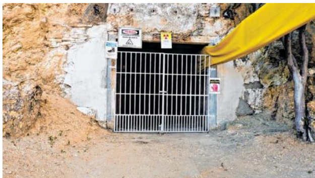
Fig.3: Main entrance to the Itataia mine.
