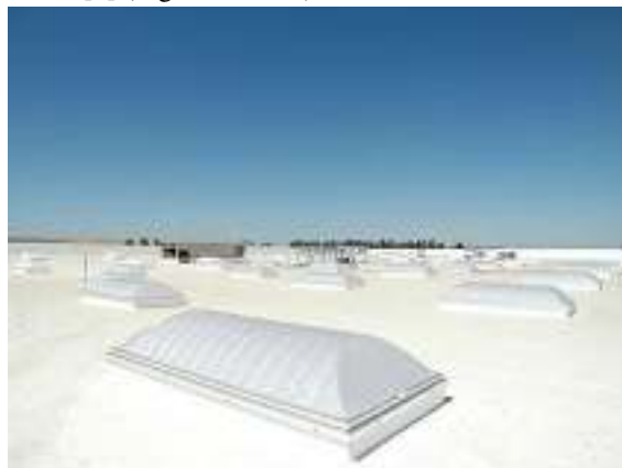
Fig.1: Installation of Prismatic Domus in the outside area.
