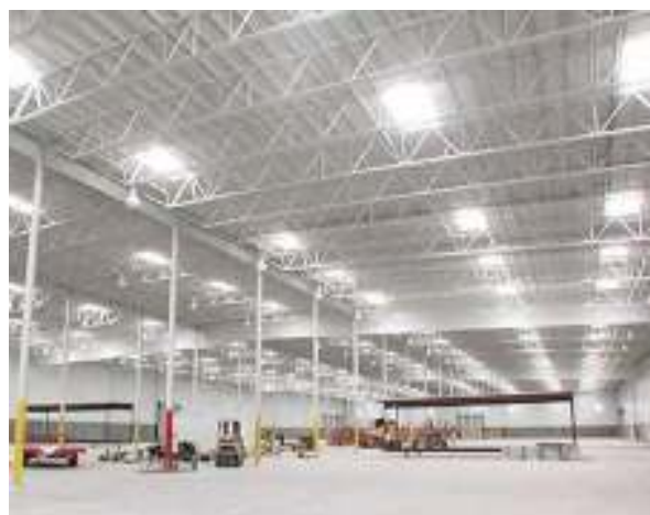
Fig.2 – Installation of prismatic domus in the inside area of the company.
