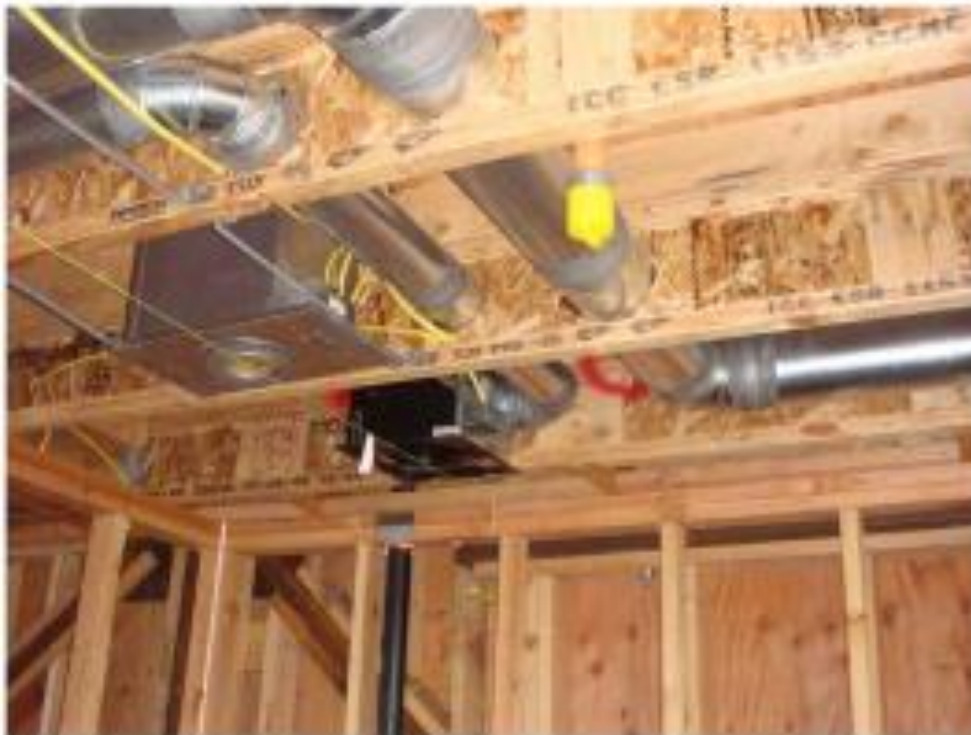
Fig. 5: Examples of Holes In Wood I-Joists, Tiberiu Polocoser, Thomas H. Miller, And Rakesh Gupta, 2013
