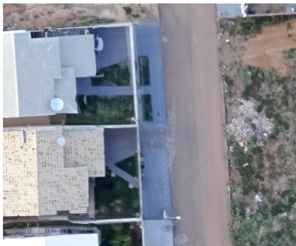
Fig.3: Painted concrete sidewalk.
