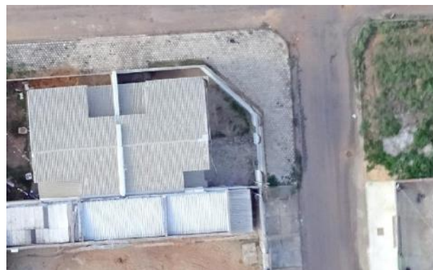
Fig.2: Detail, in mosaic, of interlocking pavers.
