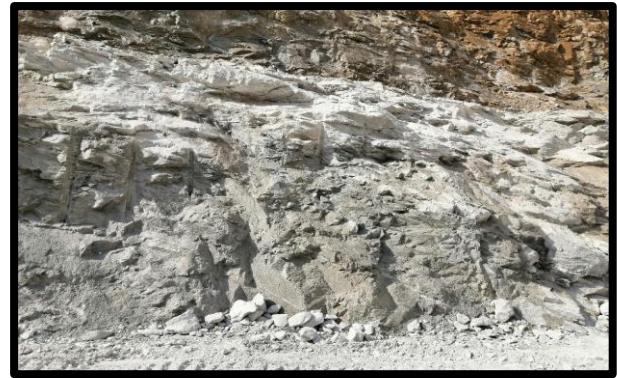
Fig.4.1: Wall Face after Wall Control Blasting
