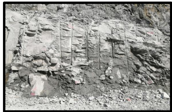
Fig.4.2: Wall Face after Wall Control Blasting
