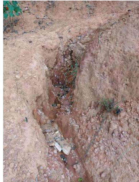
Fig.14: Erosive process caused by floods.
