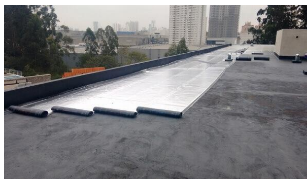
Fig.3: Waterproofing of exposed slab.
