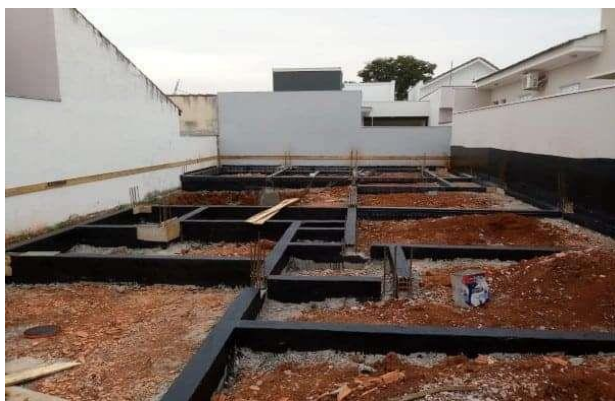
Fig.2: Waterproofed Baldrame Beam.
