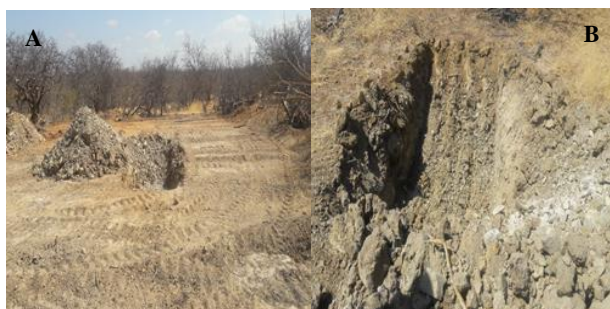
Fig.16 - Extraction of material for road burial
