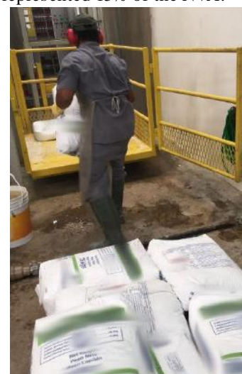
Fig. 4: sacks positioning mp1.
