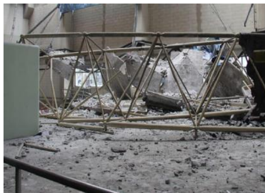
Fig. 3-5: The collapse of the scene
