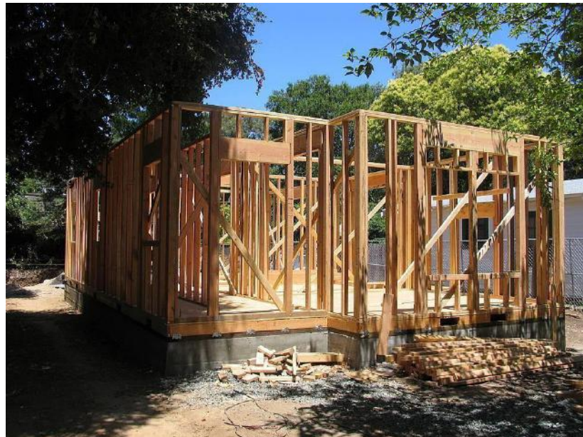
Fig.4: Wood frame construction
