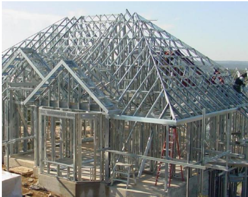
Fig.5: Steel Frame Construction
