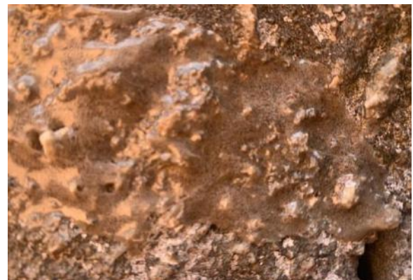
Fig 10. Thinner + Styrofoam + Kerosene on the wall
