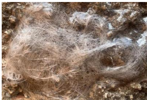
Fig 13. Thinner + Styrofoam + Fiberglass on the wall
