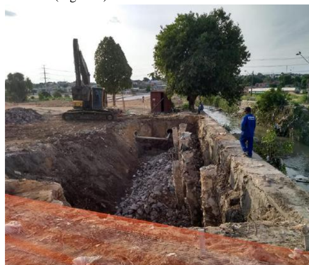
Fig. 2: Excavation for the construction of the retaining wall.
