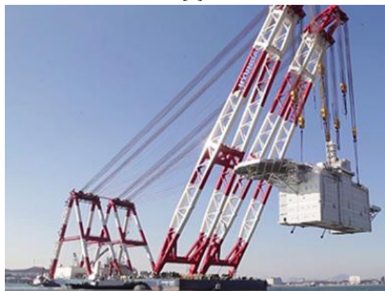
Fig.1: Rigging of a living quarter module of a platform.
